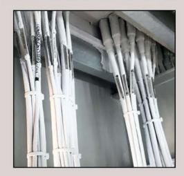
The protection time frame that Fire Security Systems Cable Coating can provide to protect electrical cables from a fire before the insulation begins to deteriorate will depend on the intensity of the flame, type and size of cables, type of insulation and other variables. In the event that a maximum time lapse protection from fire exposure is desired, a heavier coating can be applied to those areas.
